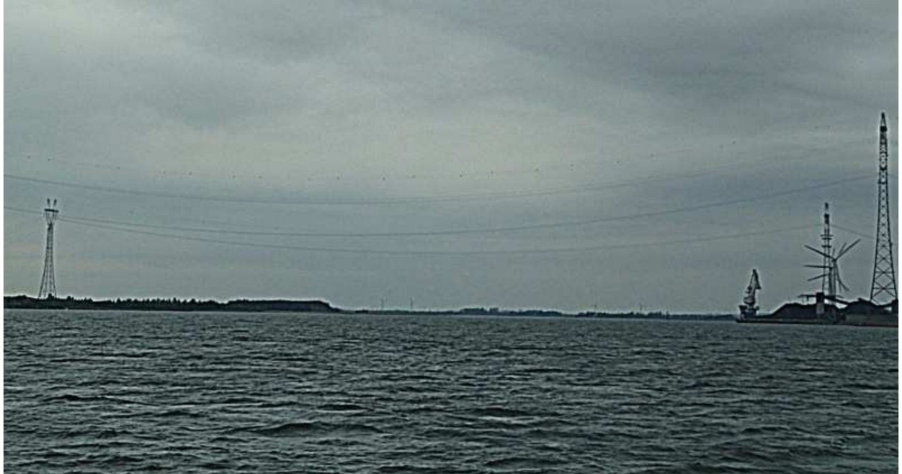
Figure 1: Transmission lines crossing Limfjorden near Nordjyllandsværket.
