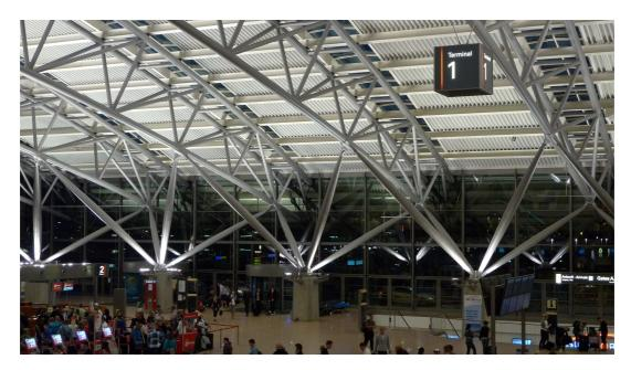
Figure 1: Truss structure support of roof in Hamburg Airport.
