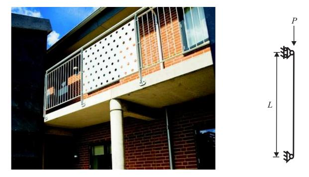
Figure 6: At left is shown a column in a real life structure and at right the corresponding static model.
